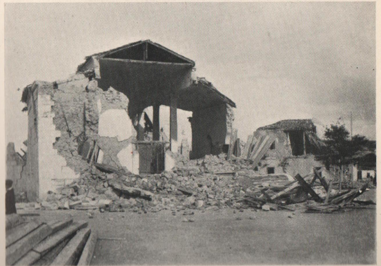
THE CHURCH OF ST. NICHOLAS, CORINTH, AFTER THE EARTHQUAKE.
